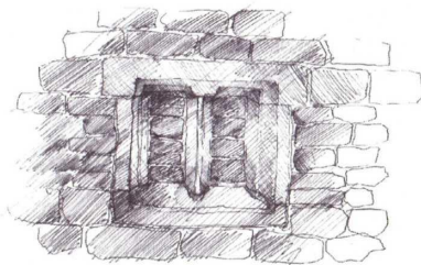
Elizabethan stone mullions in blocked up window in Back Lane
